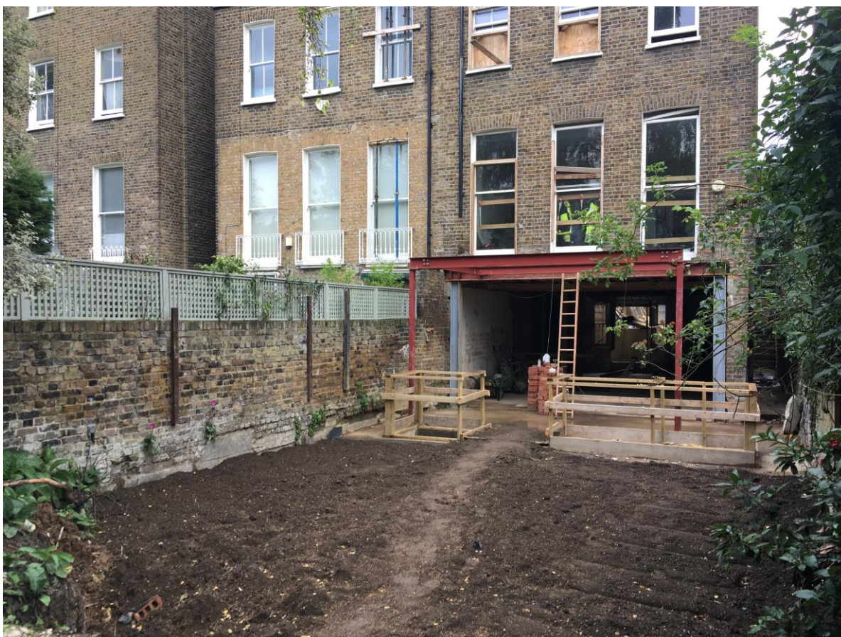
View of partially completed rear extension.
